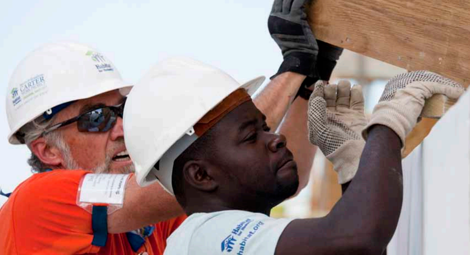
Wiline Dorcelian works alongside volunteers to help construct his Habitat house.
