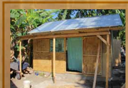
Habitat has constructed more than 1,000 upgradable shelters, which consist of a timber frame, pressure-treated plywood side walls with a permanent concrete perimeter foundation, and traditional front porch.
